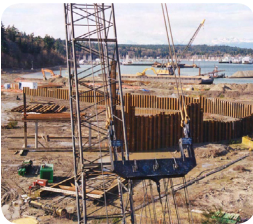
Installation of sheet piling
