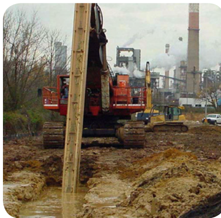
Excavation of a slurry wall trench
