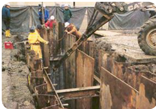
Construction of a PRB in Sunnyvale, CA
