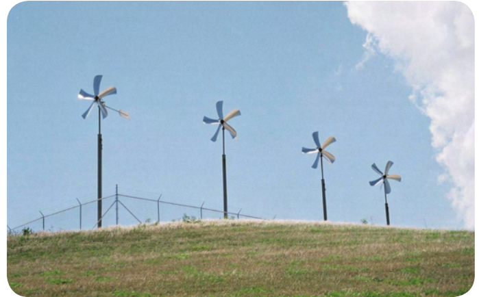
Windmills power equipment to remove oil from contaminated groundwater.
