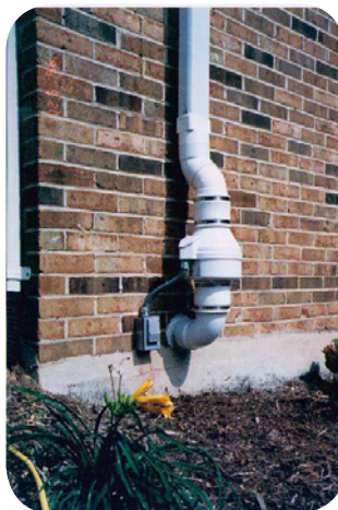
Typical fan and vent pipe.
