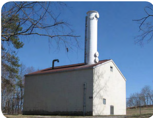
Air stripper and treatment building
