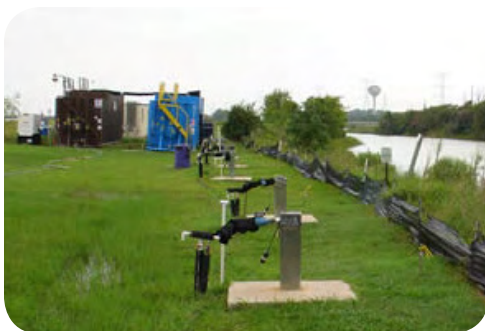
Groundwater Pumping Wells
